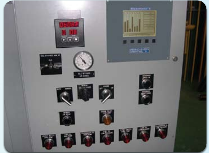
Alarm Monitoring with ConsoliDator
