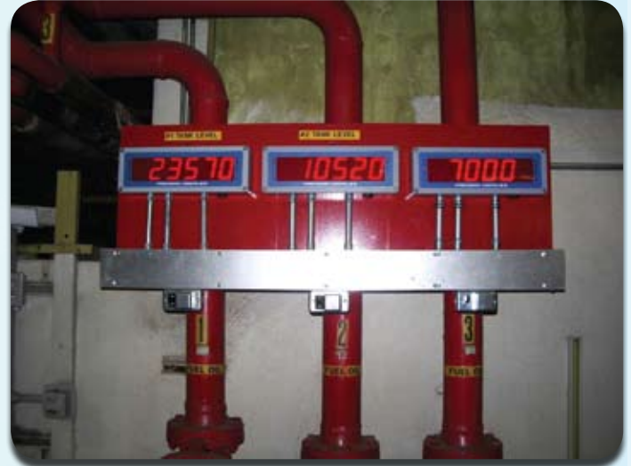
Tank Level Monitoring with PD650
